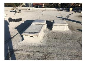
New Roof Openings & Insulation for HVAC Duct
