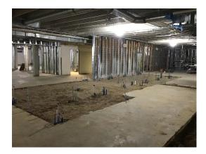
Backfill for Underground Plumbing at Dental Lab
