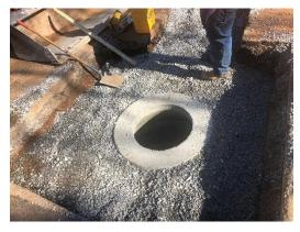
Stone Backfill at Sanitary Sewer Tie-In
